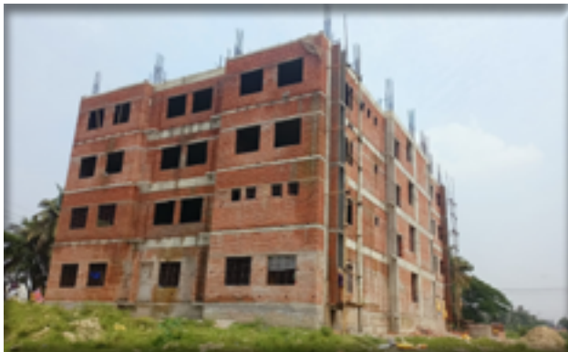
Construction works of JBF hospital at Laksham, cumilla is going on
