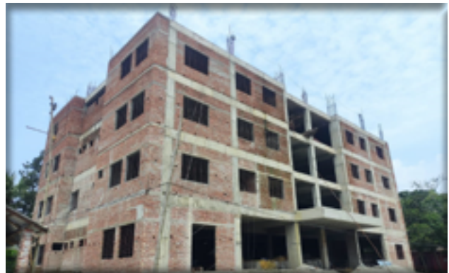
Construction works of JBF hospital at Barura, cumilla is going on
