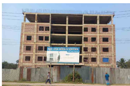
Construction works of JBF Hospital at Rupgonj, Narayanganj is going on
