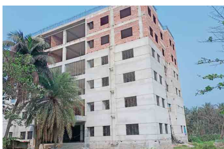
Construction works of JBF Hospital at Laksham, Cumilla is going on
