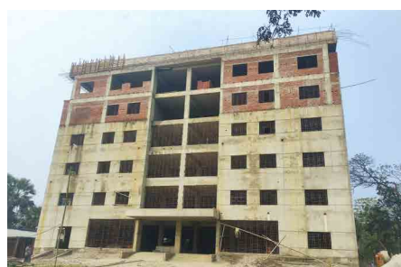
Construction works of JBF Hospital at Barura, Cumilla is going on
