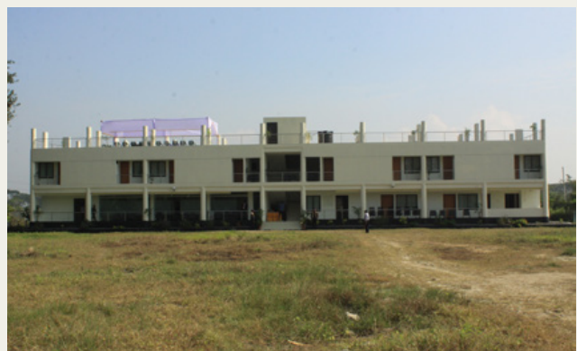
Newly constructed 2(two) storied building of old home
